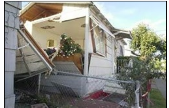
Home destroyed by TRF explosion San Diego, 1992
